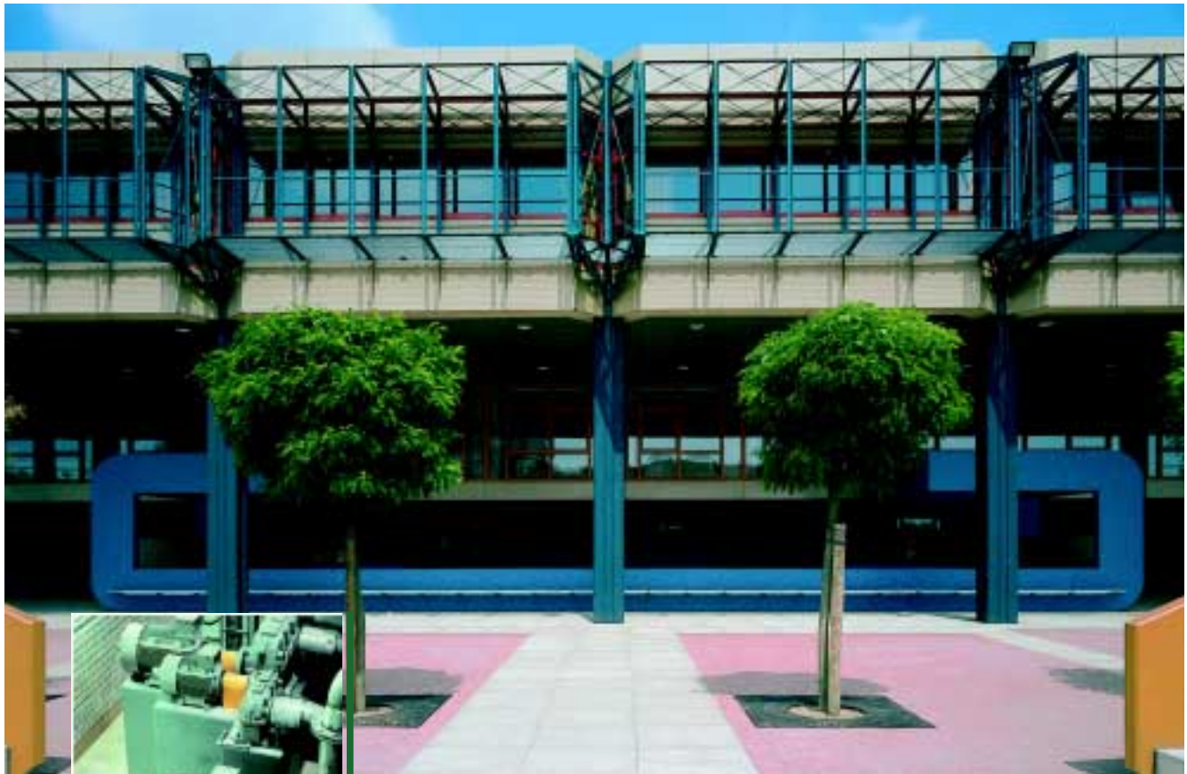
Energy saving: A low maintenance, highly efficient system of 150 heat pumps generates the optimal "educational climate" in a school. POG 9 Digital-Tachos from HÜBNER are incorporated in the speed control system for the asynchronous motors.
