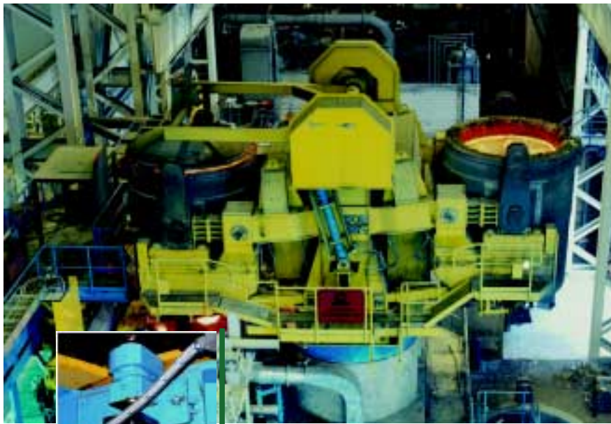
Linear measurement and smooth running: In this continuous casting plant, AMG 10 absolute multiturn encoders and water-cooled POG 10 Digital-Tachos provide the signals for the feed speed and the length of the items produced.
