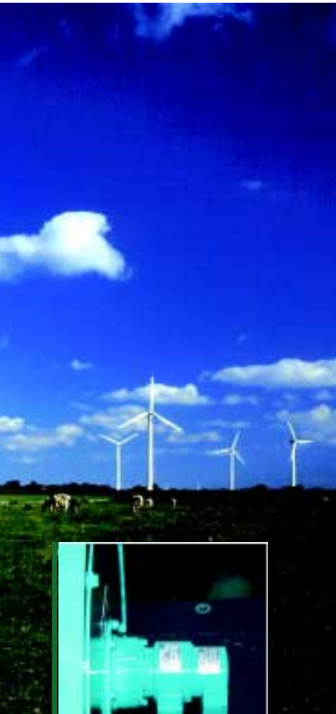
Wind power under control: POG 90 + FSL, combinations of Digital-Tacho and mechanical rotational speed switch, control and monitor the speed of 1.5 MW wind power generators.
